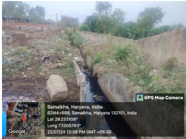
Figure 5: Drain no. 6 near Samalkha, Panipat
